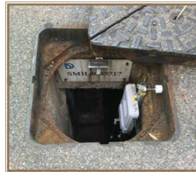
An Integrated Sensor Module and Ubiquitous Wireless Network for Smart Drainage System 結合無線傳感模組及網絡的智能渠道管理系統
